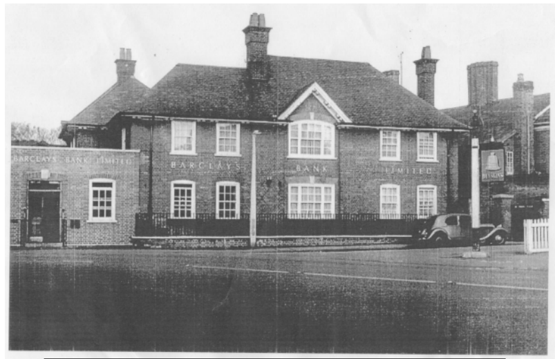
BARCLAYS BANK HATFIELD BRANCH AT FORE STREET
